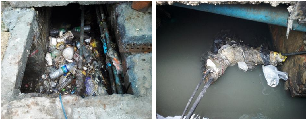
Figure 2.5 Sediments in the drain and sediment dredging work
