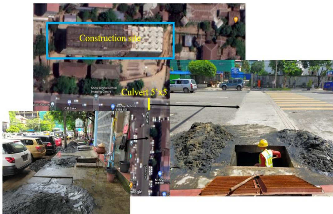
Figure 7.10 Construction material extracted from the drainage (source-DWA Latha)
