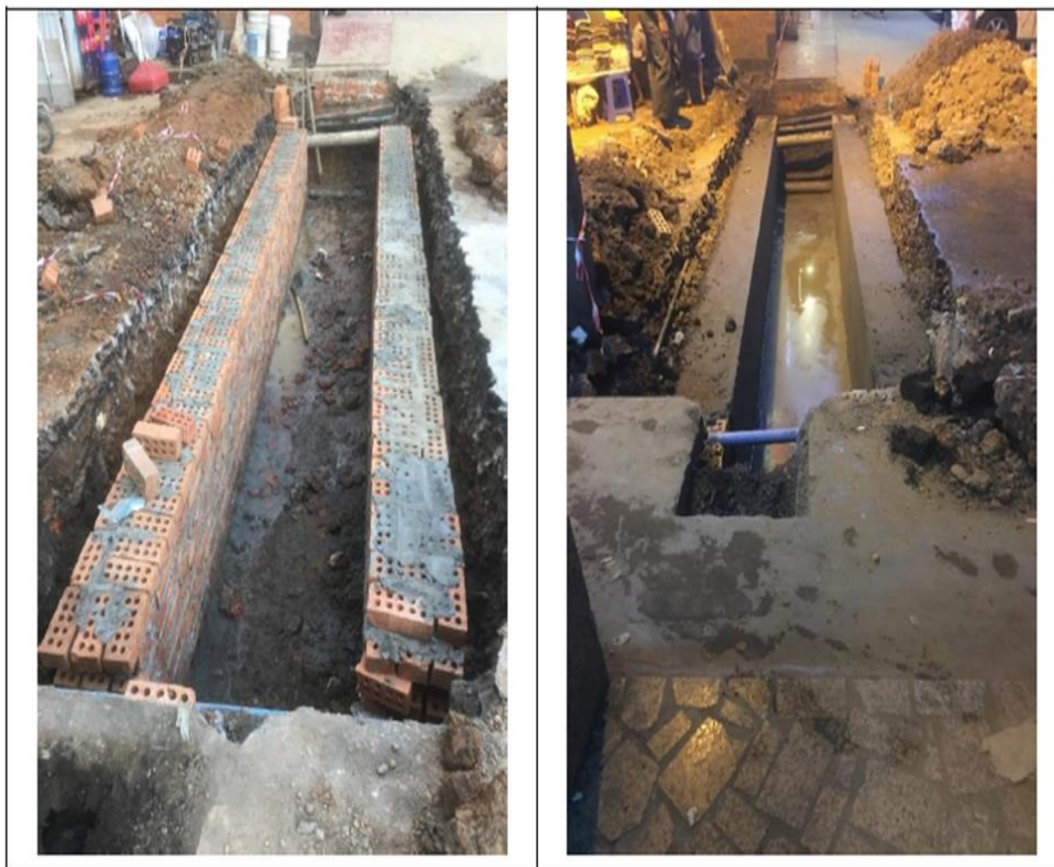
Figure 7.12 Cross road culvert 31 st street under construction February 2019
