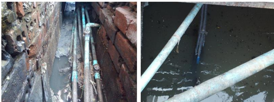
Figure 7.7 Utilities pipes and cables existence in Yangon drain (source-DWMA Latha)
