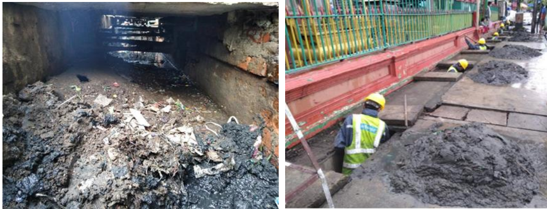
Figure 2.5 Sediments in the drain and sediment dredging work
