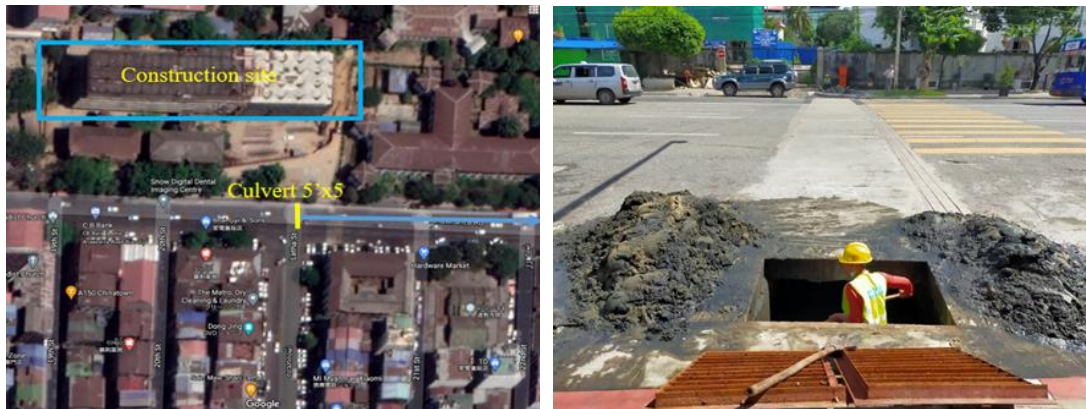
Figure 2.8 Sediment blockage due to construction materials in the drain
